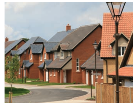
Balfour Beatty redevelopment at RAF Lakenheath
